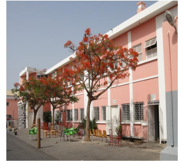
Praia Center Hospital in the Republic of Cape Verde
