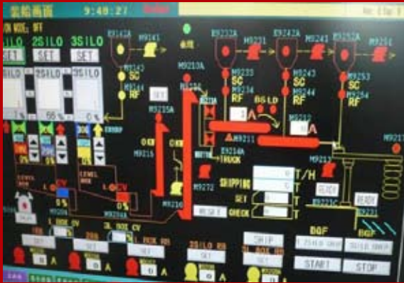
Qingdao port cement storage project
