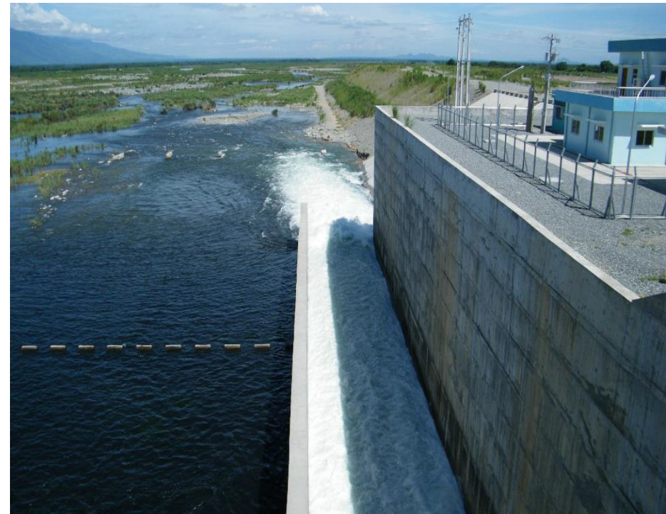
Scouring Sluice at Weir-left Side
