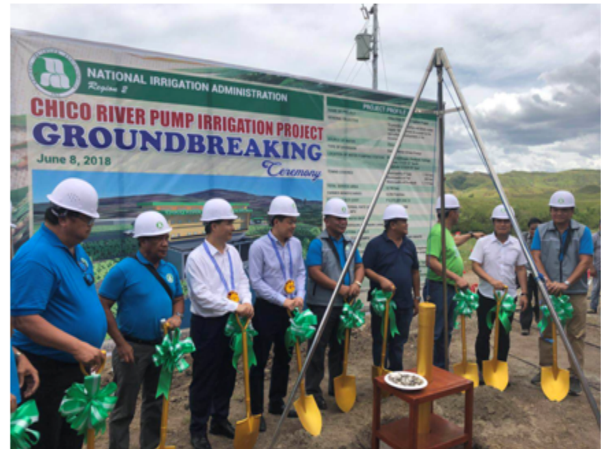
Ground Breaking Ceremony
