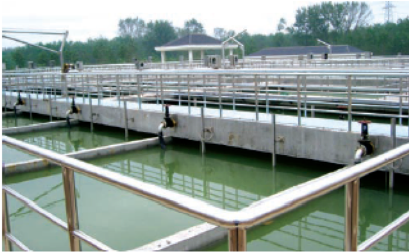
城北污水处理厂项目生化池内景 Interior of the Biochemical Tank of Chengbei Waste Water Treatment Plant
