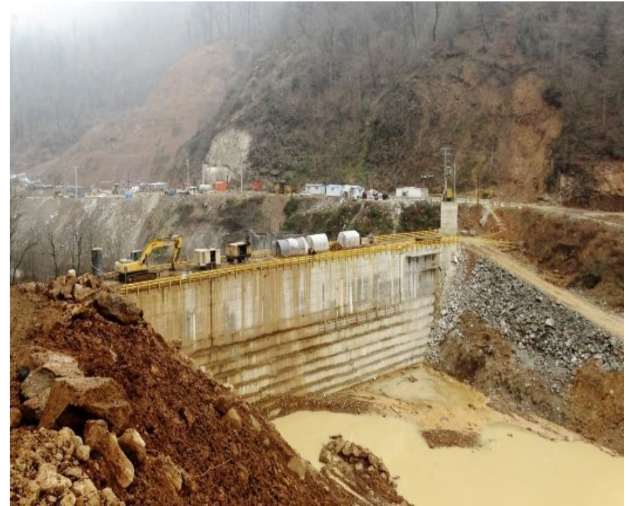
Concrete dam construction
