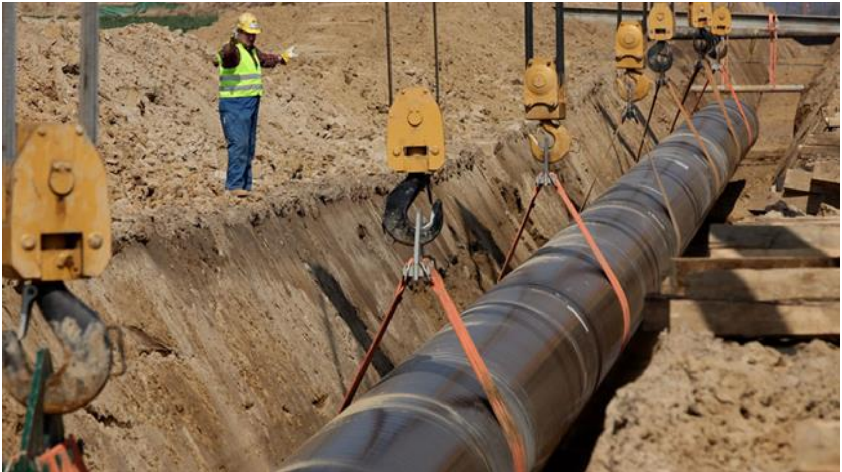
Water Pipe Under Installation
