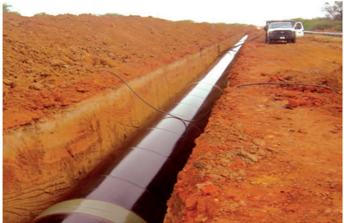
Water Pipe on Installation
